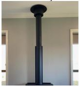
The <u>FULL</u> RSF flue kit has the insulated flue starting directly on top of the fire. You can only use this style if the heater was tested with this configuration.
